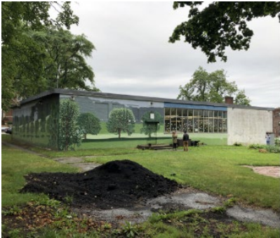
Rear of Building
